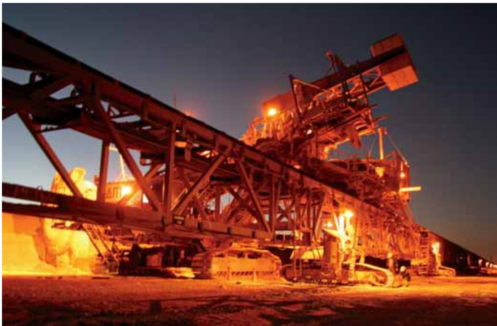
The reclaim conveyor at the leach pad operates around the clock at the Zaldívar copper mine in Chile.
