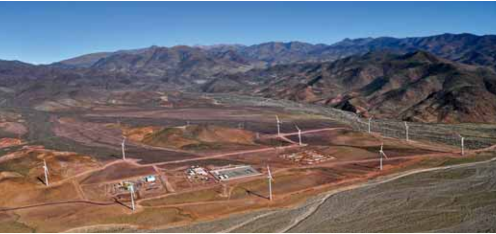
Barrick's $50 million Punta Colorada wind farm in northern Chile is the largest ever built by a mining company in the country. It consists of 10 turbines that generate 20 megawatts of power.
